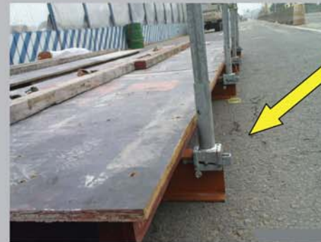
Viaduct cat walk guide rail clamp EZ03.
